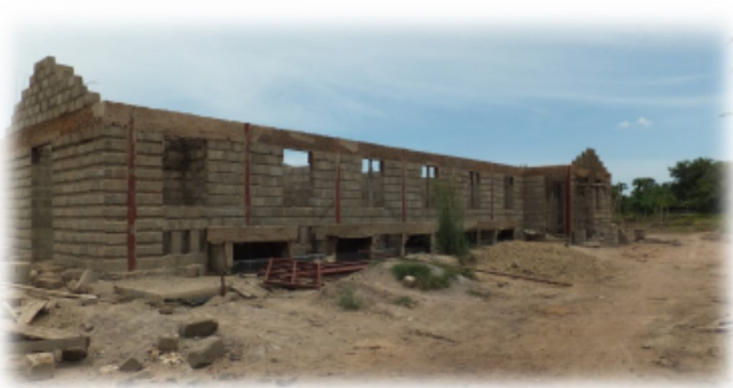
New dormitory under construction
